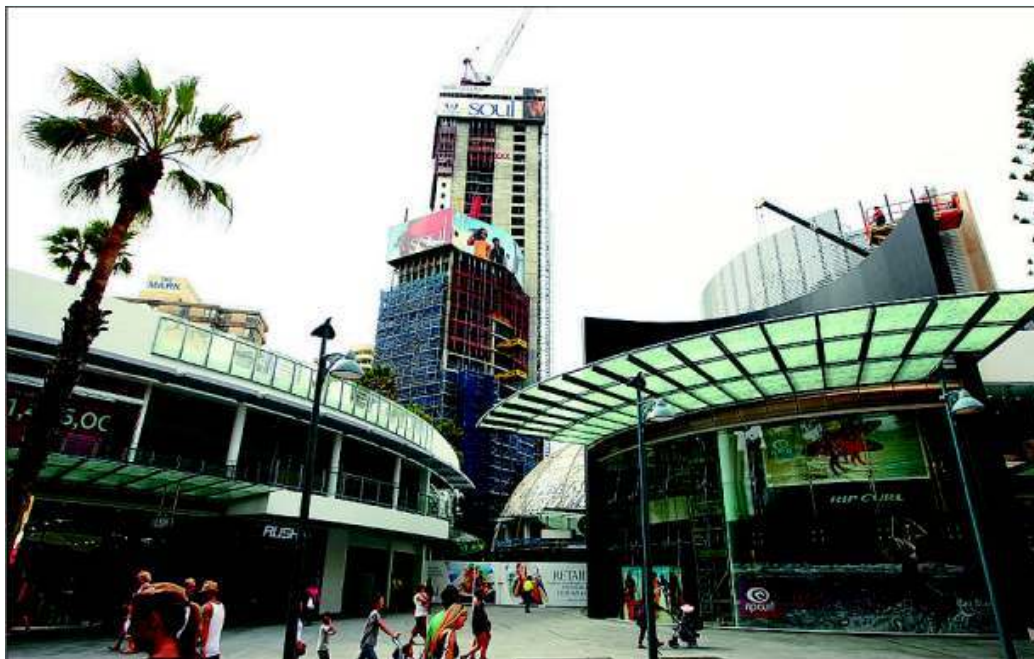
The retail strip under Soul is growing with new outlets opening regularly
